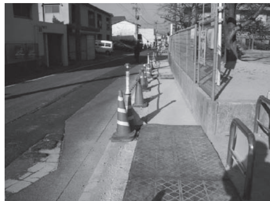
Photo 1 Sidewalk installation work
